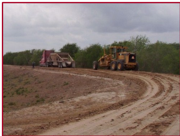
Lower Rio Grande Levee
